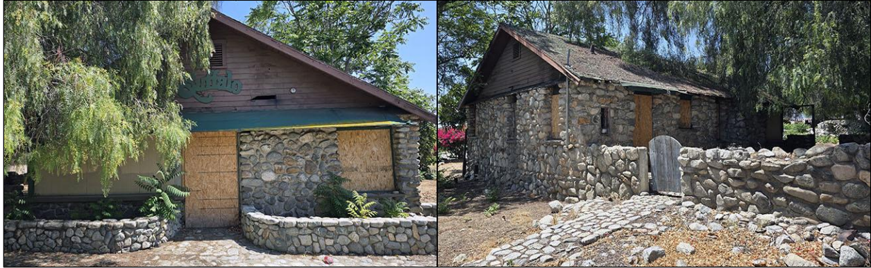
Building A, residence at 1814 W. Foothill Boulevard. Left: front façade, view to the south; right: rear façade, eastern façade, and side courtyard, view to the northwest
