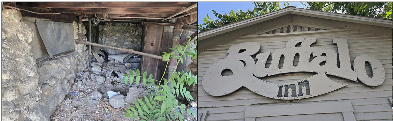
Building E, residence at western end. Left: crawlspace entrance, view to the east; right: Buffalo Inn sign above front door, view to the south
